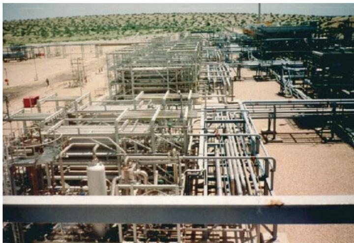
**Figure 8.10** Photograph of the 500-million scfd CO<sub>2</sub> removal plant installed by UOP at Kandawari, Pakistan. The UOP Separex system reduces CO<sub>2</sub> content of a natural-gas stream from 6.5 to 2% CO<sub>2</sub>. Photo used courtesy of UOP, LLC.
